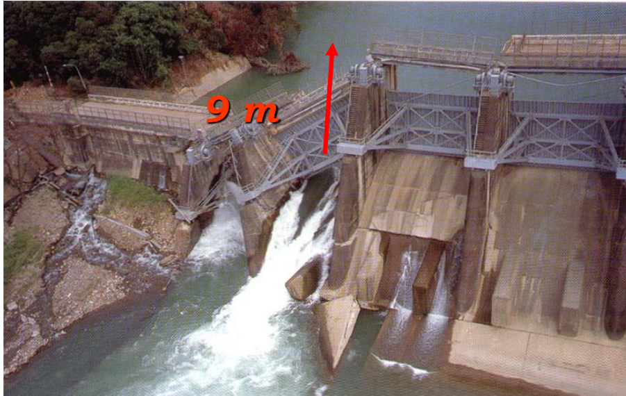
Fig. 4.4.1 Example of a fault disruption at Shih-Kang dam during the Chi-Chi earthquake in Taiwan (1999) ( Courtesy of Prof. Gazetas )
