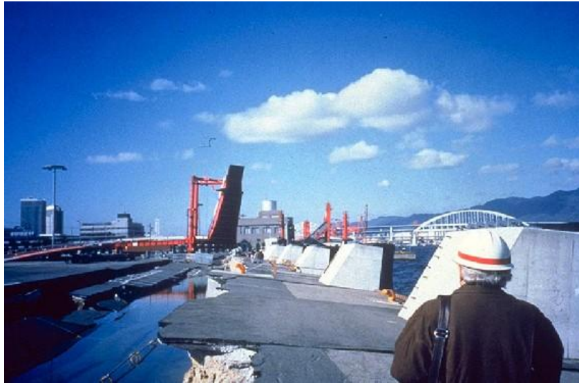
Fig. 4.7.1 Example of soil liquefaction behind a retaining structure (Kobe, 1995)
